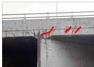
Figure 6. Cracks in the slab above the pillars
