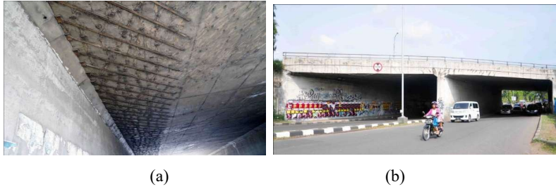
Figure 2.a. Cracks on the underside of abutment; 2.b. Cracks on the upper-side of pillars
