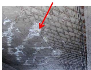
Figure 5. Cracks on the slab that has penetrated all the way to the bottom
