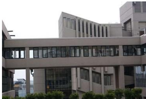
Figure 4. Independent Structure Skybridge at University of Leeds, Ohio
