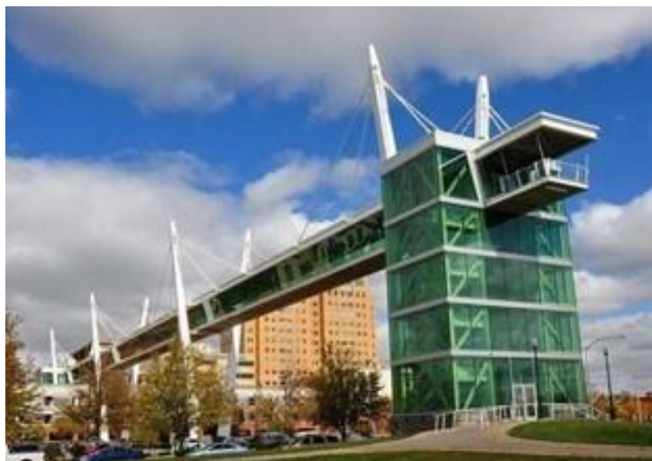
Figure 5. Semi-Independent Skybridge in Davenport, USA
