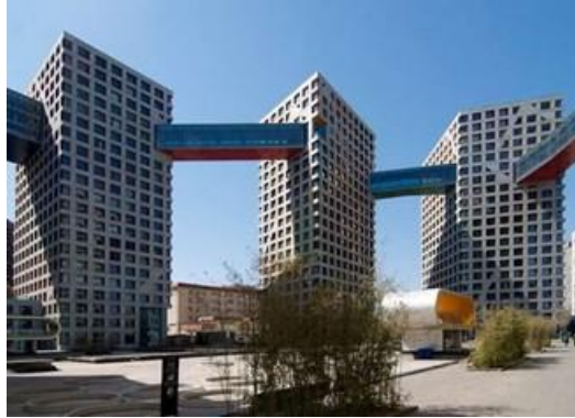
Figure 3. Attached Skybridge at Linked Hybrid, Beijing, China
